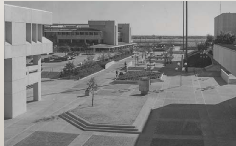
This archival photo lends credence to the “concrete canyon” description of the mall prior to renovation.
